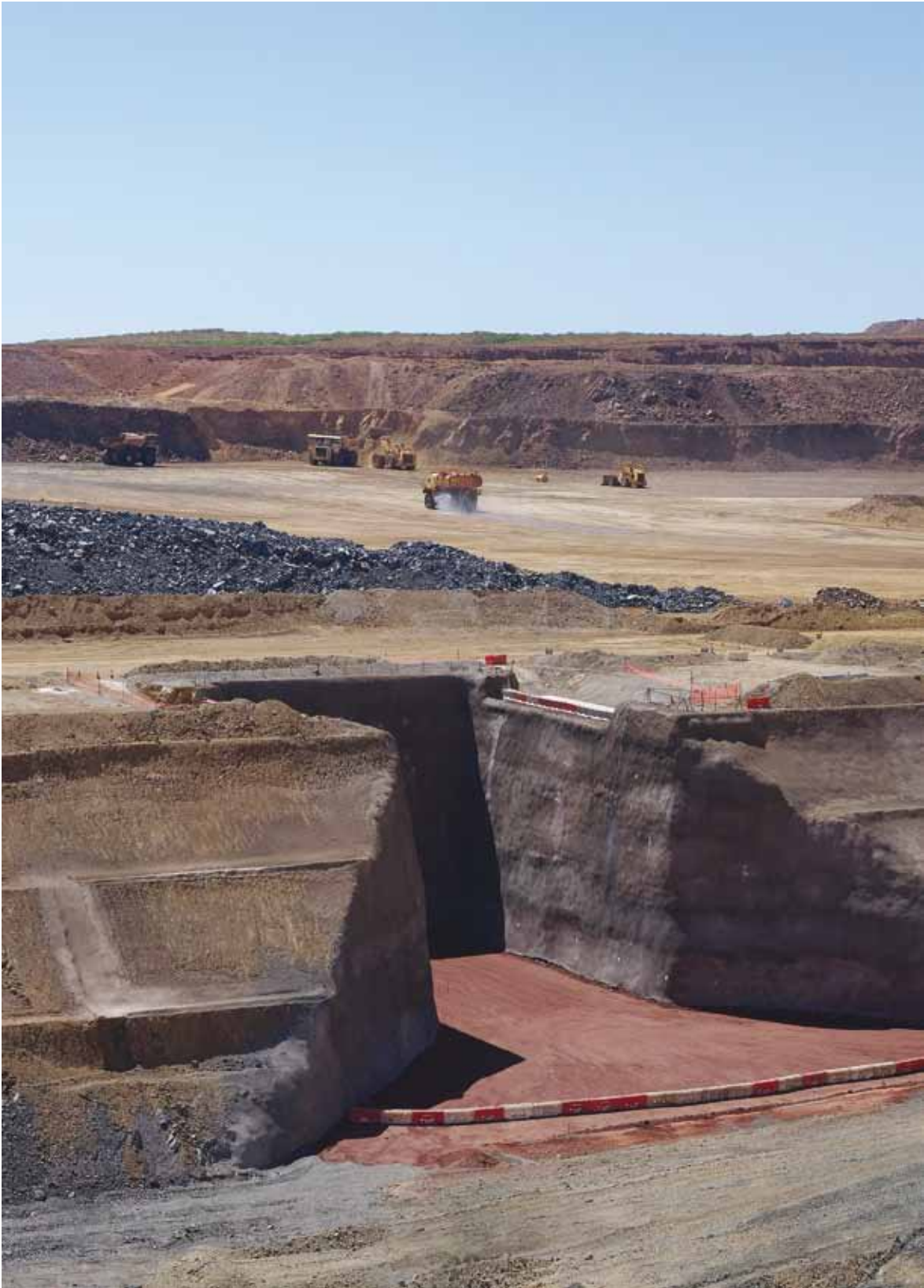
One of four crusher slots at CITIC Pacific Mining’s Sino Iron Project in Western Australia’s Pilbara. Photo courtesy of CITIC Pacific Mining.
